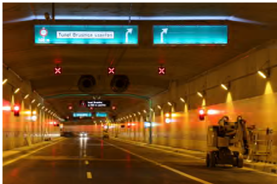
The northern cut-and-cover tunnel under Milady Horákové Street near Špejchar (photo by Jakub Karlíček)
